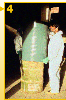
4 Old barrels are stored in the outer UN barrels.
